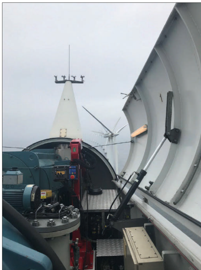
Figure: the right hatch is open. Note the mechanical lock system to be opened before opening and locked after closing.
